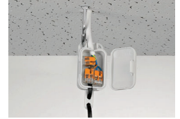
Pendant light connection in a suspended ceiling
