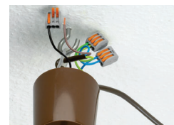
Lighting fixture connection with fine-stranded wires and power feed
